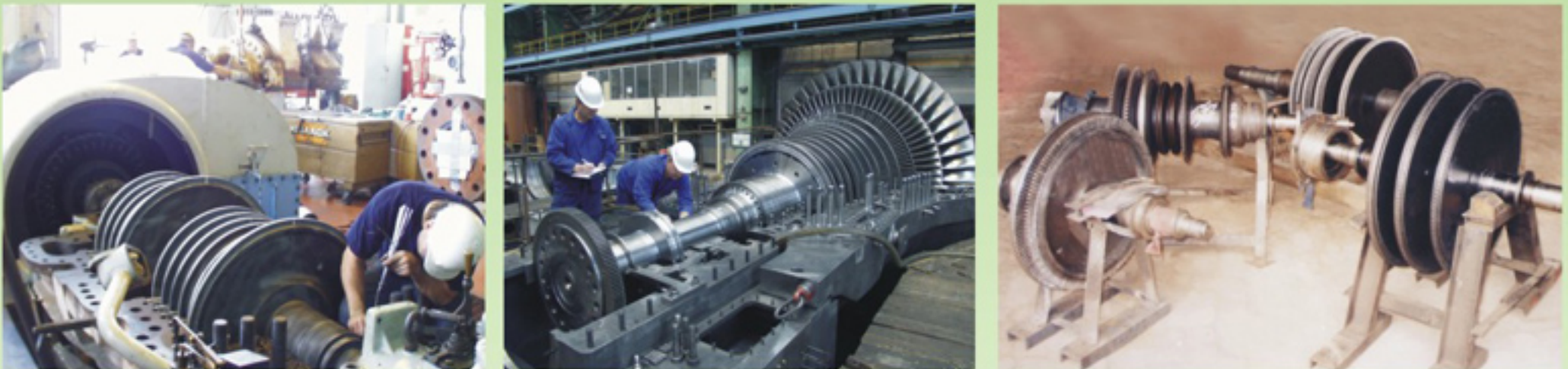
Energy Plant Power House and Mill House turbine alignment process
